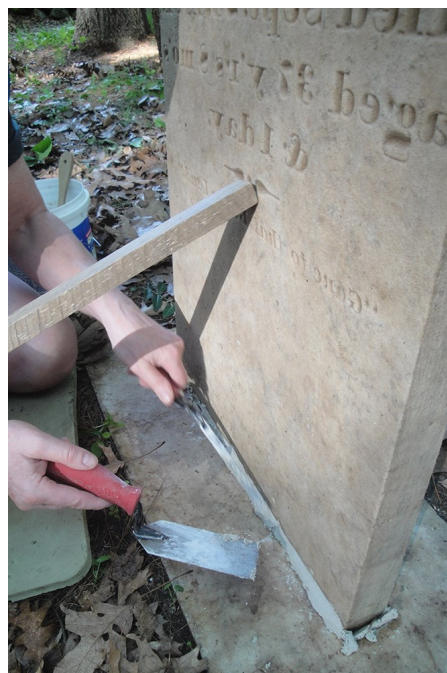
Applying high lime mortar inside slot of a base. Cemetery #29, Burrillville
