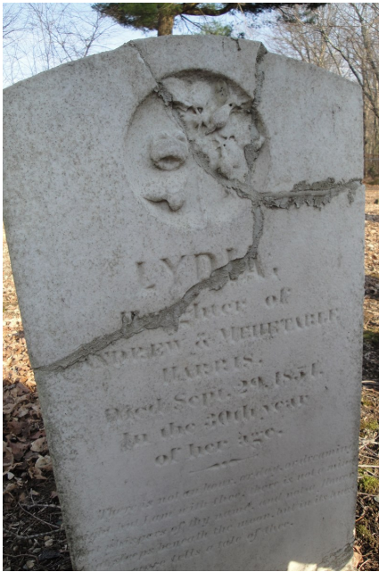
Use of hard Portland mortar to repair broken stone. Careless application obliterates some of the inscription. It is impossible to repair this stone correctly because this Portland mortar can NEVER be removed!
