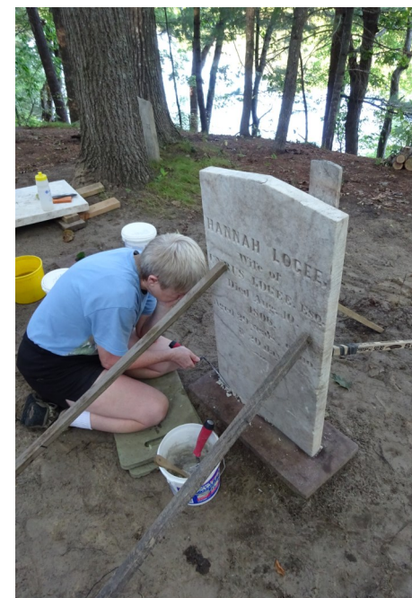
Applying high lime mortar to fasten gravestone to base. Cemetery #93
