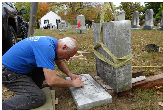
4. Monument compound is applied to base.
