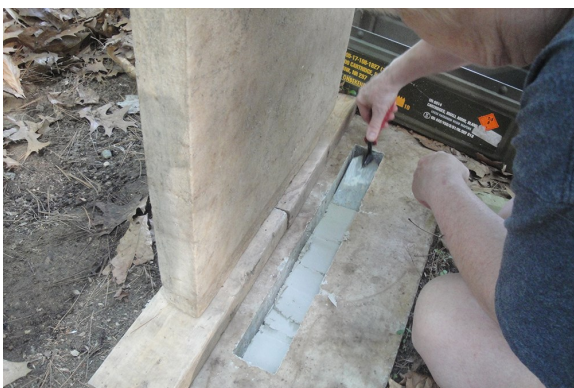
Applying high lime mortar inside slot of a base. Cemetery #29, Burrillville
