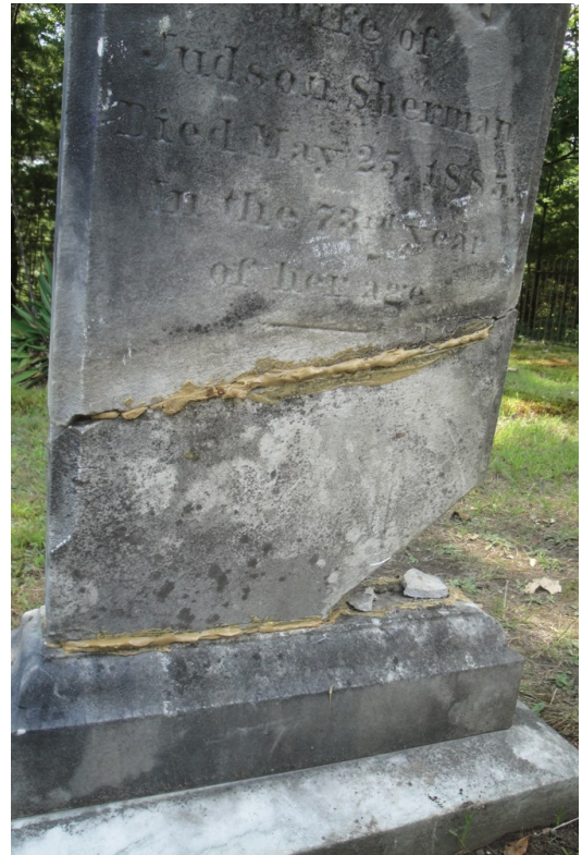
Unskillful use of caulks that don't adhere properly and repair fails,
